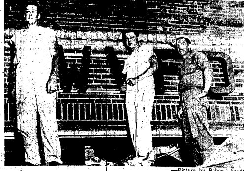
Wayne firemen installed new metal identification letters on the face of the city hall this week. The metal WVPD represents Wayne Volunteer Fire department. Pictured above installing the letters are, left to right, Earle Koskovich, Doug Crain and Lee Swinney.
